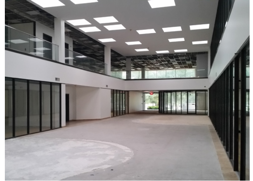
CLEAN SHELL CONDITION
